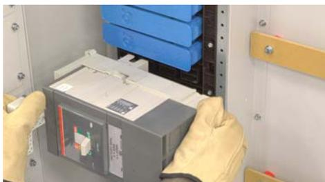
The Breaker Is Inserted Into The SafePanel
