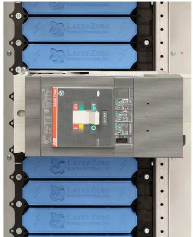
**Type-S 1200 A Circuit Breaker Installation Process**
